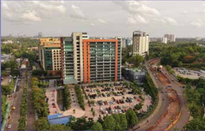
Construction is underway for Kochi Metro Rail Ltd's Phase 2 line, passing Infopark.
